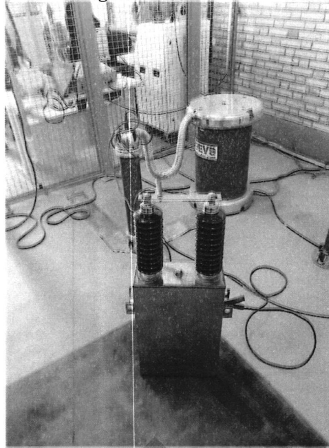
Figure 3: AC voltage test between terminals and container
