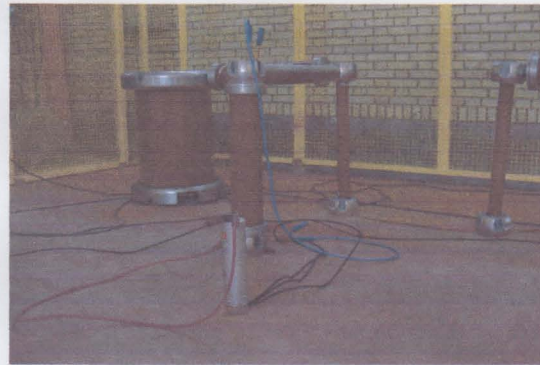
Figure 3: Voltage test between terminals and container
